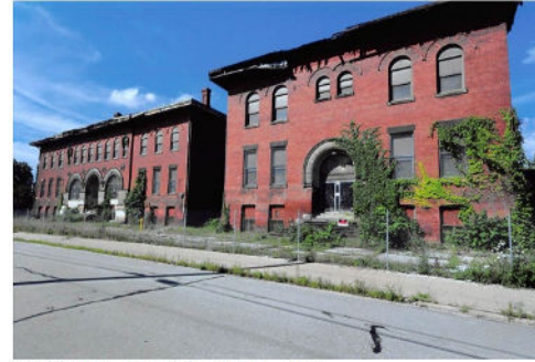
WINSLOW ST - LOOKING NORTH - 2015
