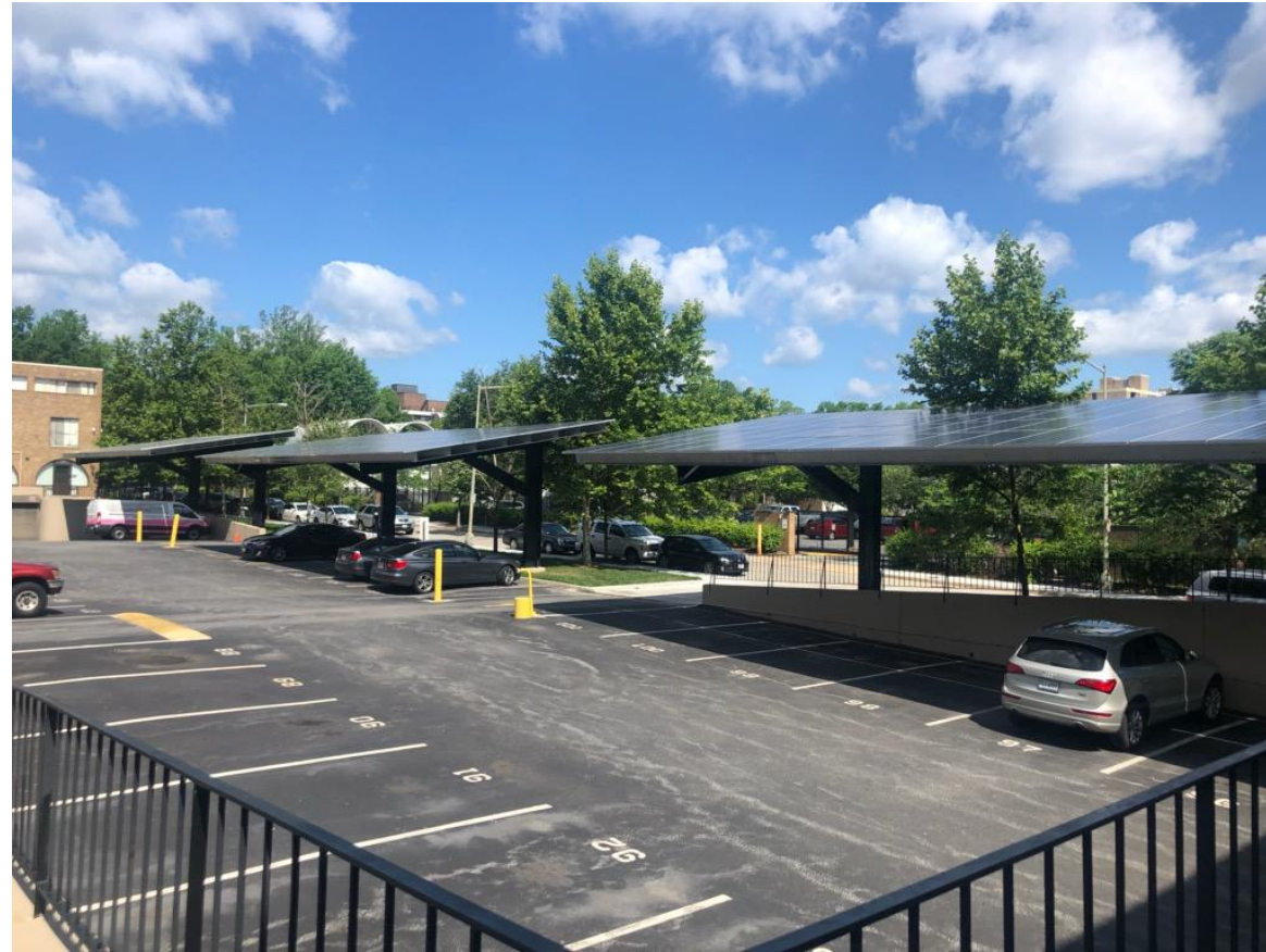
Channel Square Apartments Washington, D.C.
