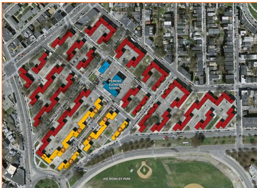
site aerial pre-construction
