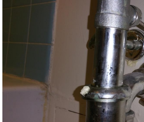
Air-Sealing Pipe Penetrations
